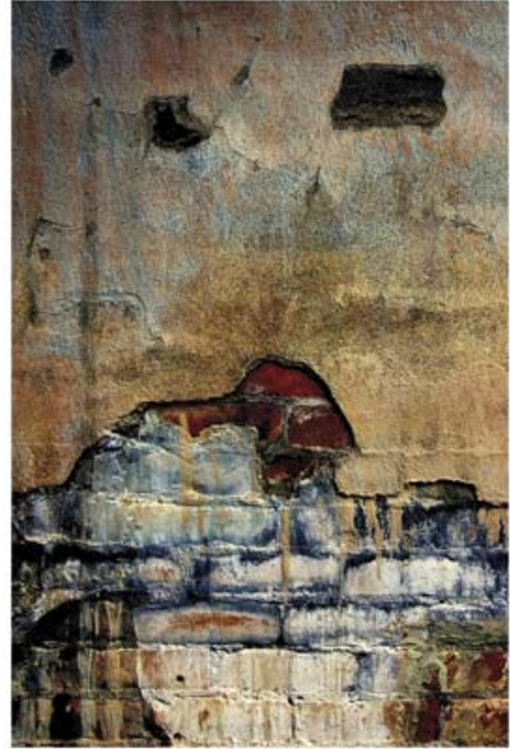
Time Well Worn - TR15172
